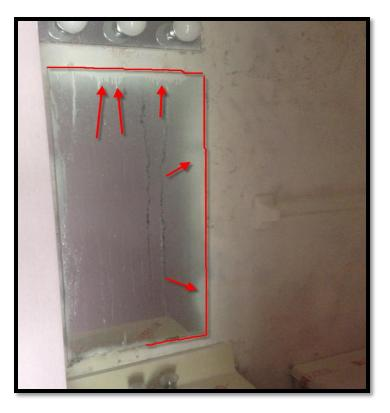
Close up photo showing <u>paint runs</u> on the bathroom mirror. Notice the poor and uneven and thin coverage of the sealed surfaces.
