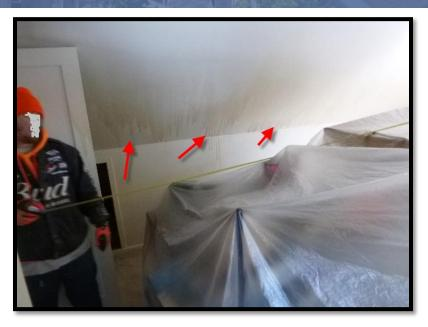
Arrows point to clear lines where the discoloration has begun to appear. This is early stage low density discoloration treatable with "Treat and Seal". A painter's drop cloth is to be used to protect carpet when sealing with appropriate primer.
