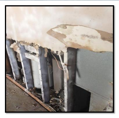
Wall board is to be cut with a saw or removed at a factory seam to perform a professional demolition service so no additional demolition is required by the renovation contractor.
