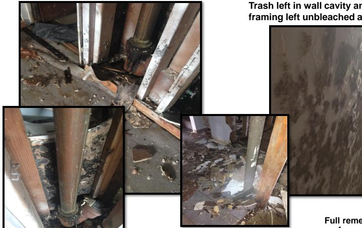
Trash left in wall cavity and on floor. Wall framing left unbleached and unsealed.
