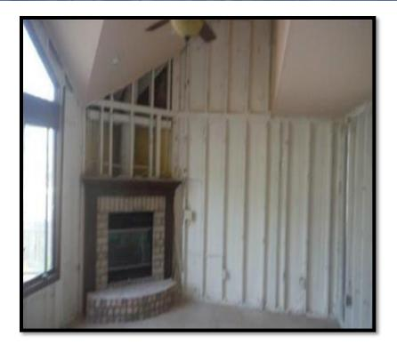
Vendor did a nice job of sealing the wall cavity discoloration but only applied one coat without prior bleaching.
