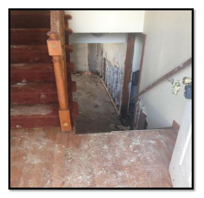
Typically, the bottom four feet of basement walls often are removed when heavy density discoloration is present. Notice the hardwood floor unprotected during the drywall demolition and left unclean.
