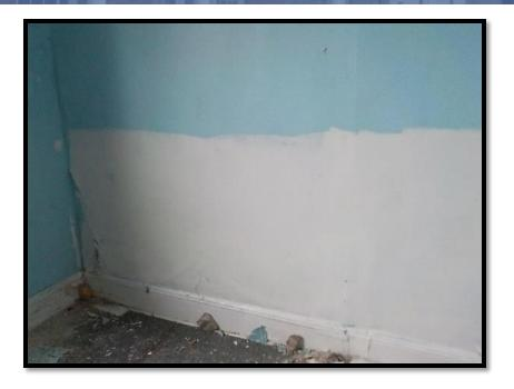
This photo shows the bottom 3 feet of the wall sealed in a close up view of the corner of the room which is good.
