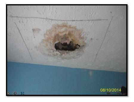
Ceiling damaged from roof leak causing the start of discoloration.
