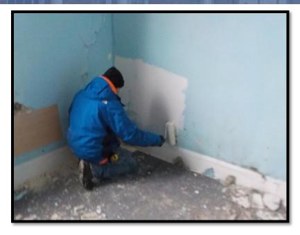
Application of sealer is to be performed on dry wall board after the spore kill has been address through previous antimicrobial spraying. Brush or roll sealer, DO NOT use aerosol spray cans.
