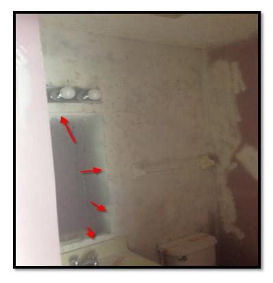
Vendor <u>used spray cans</u> and unprofessionally sprayed across edges of mirror without protecting.
