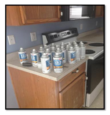
Vendor <u>incorrectly used spray cans</u> instead of roller and brush thereby not providing a thick enough coating to properly seal discoloration (only hide it).
